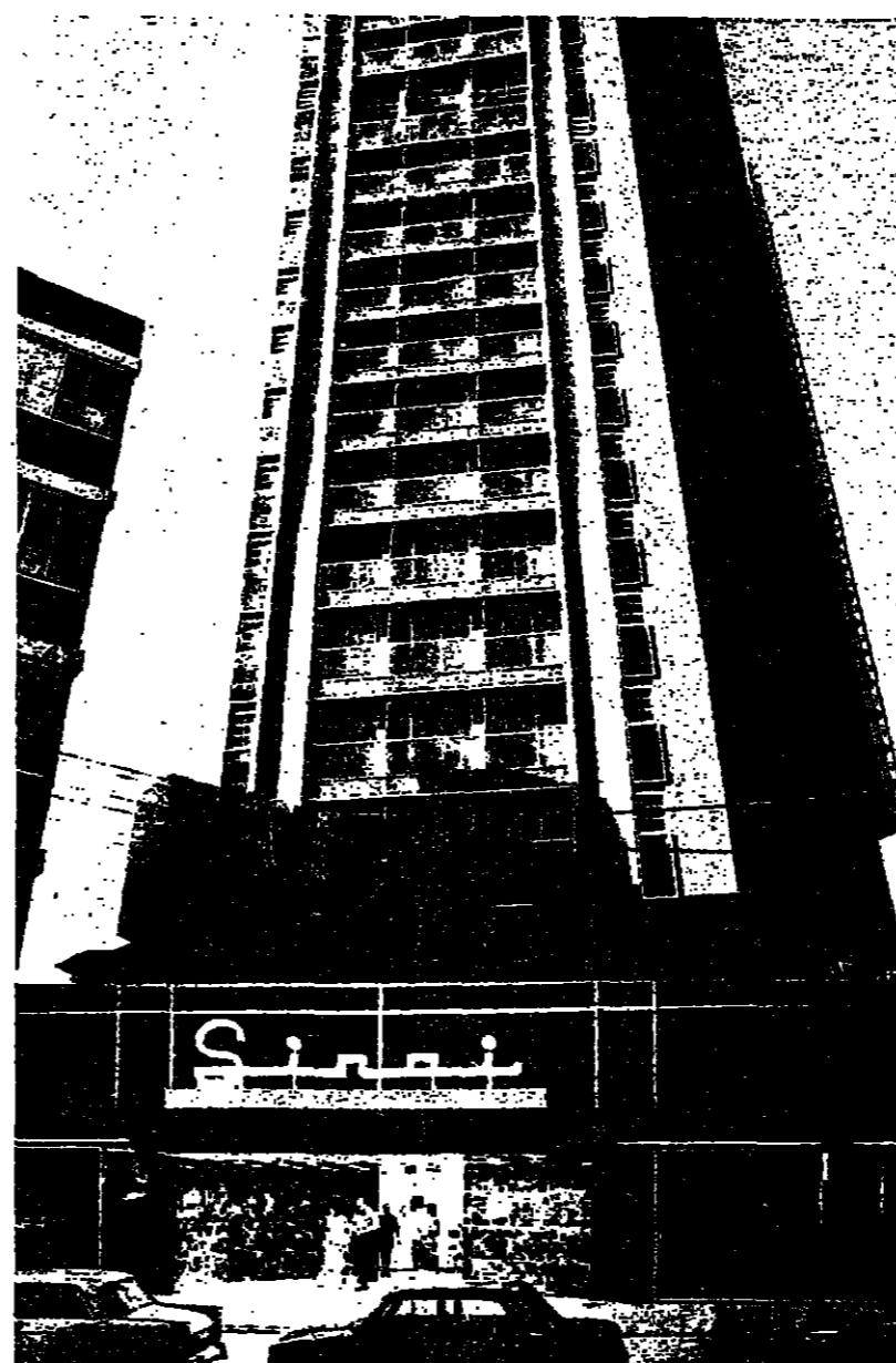
Tel Aviv's Sinal hotel makes maximum use of its limited space.
